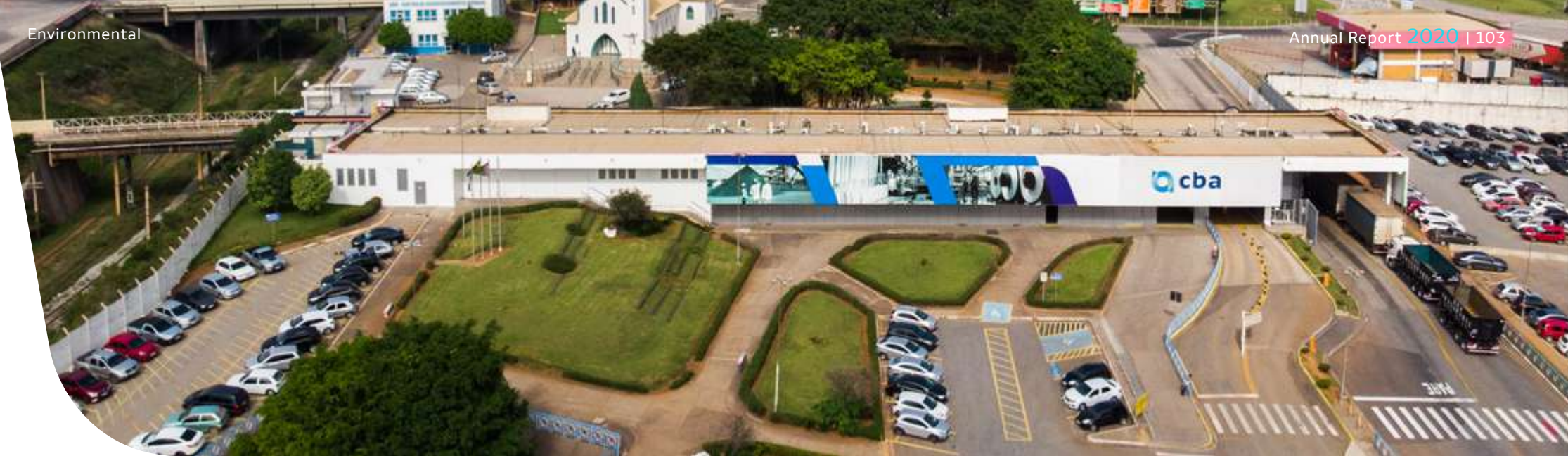
The facade of the Aluminio plant
