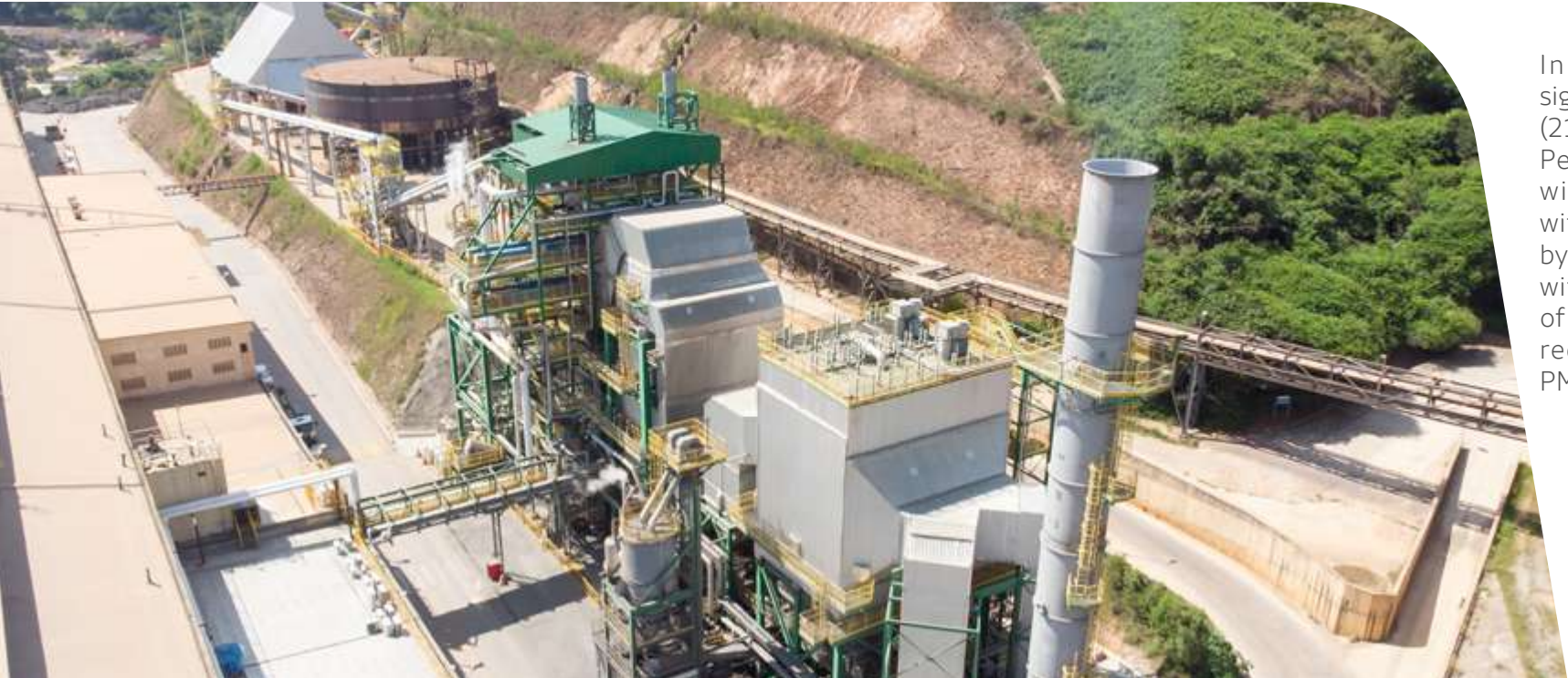
A biomass boiler to produce steam at the Alumina department
